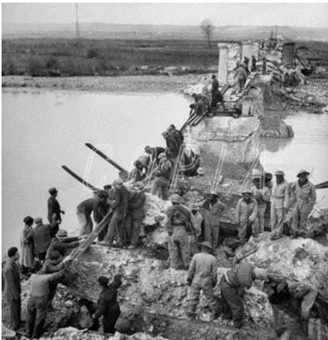
Sangro Bridge being built by Africans and Italians
