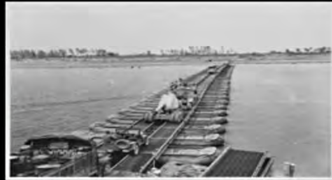
Convoy Crossing River Po on a Pontoon Bridge, April 1944
